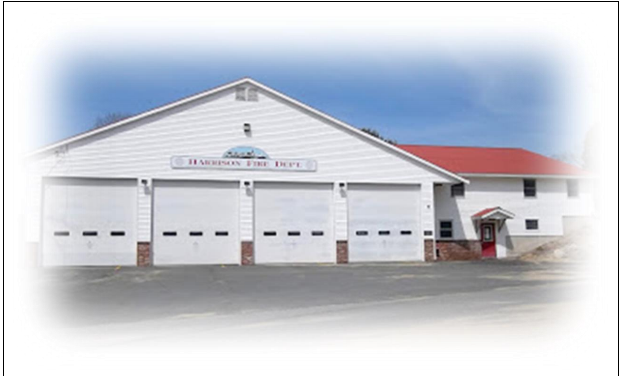
Figure 7 – Harrison Fire Station 34 School Street, Harrison, Maine
