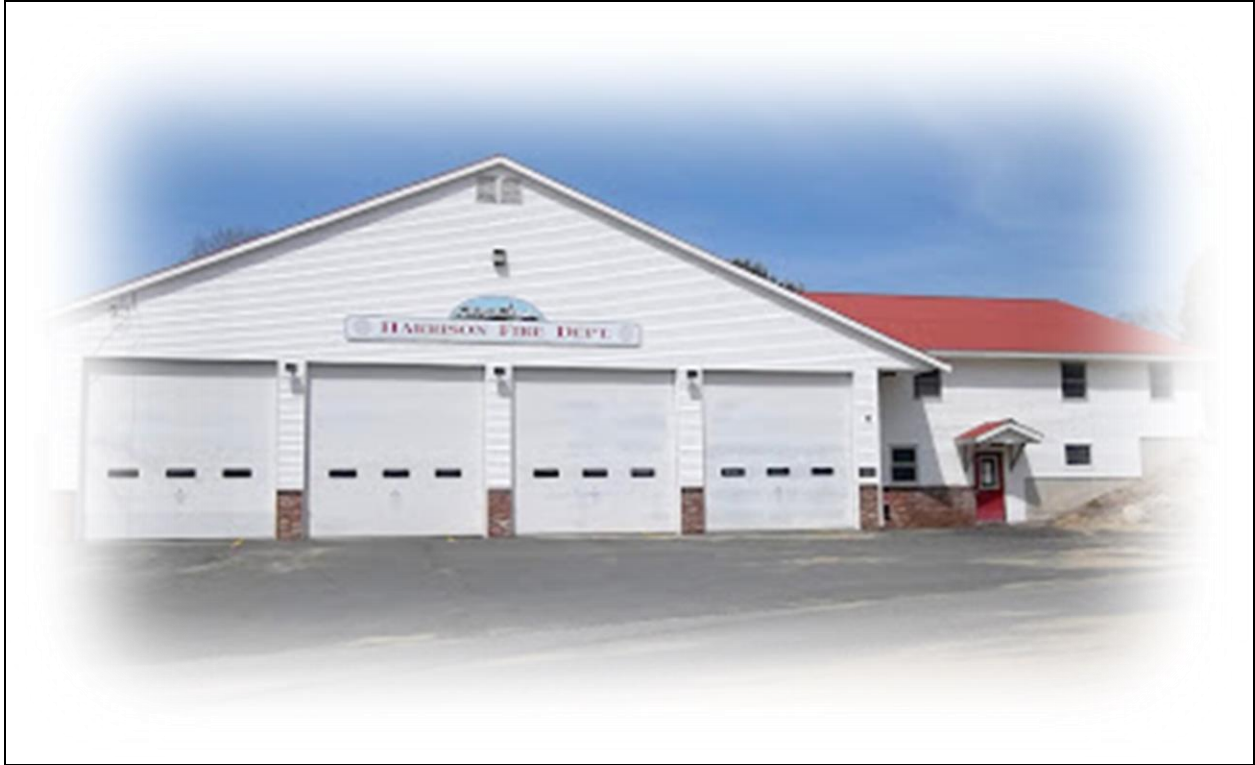
Figure 7 – Harrison Fire Station 34 School Street, Harrison, Maine
